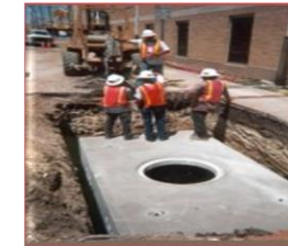
Underground Utility Vaults
