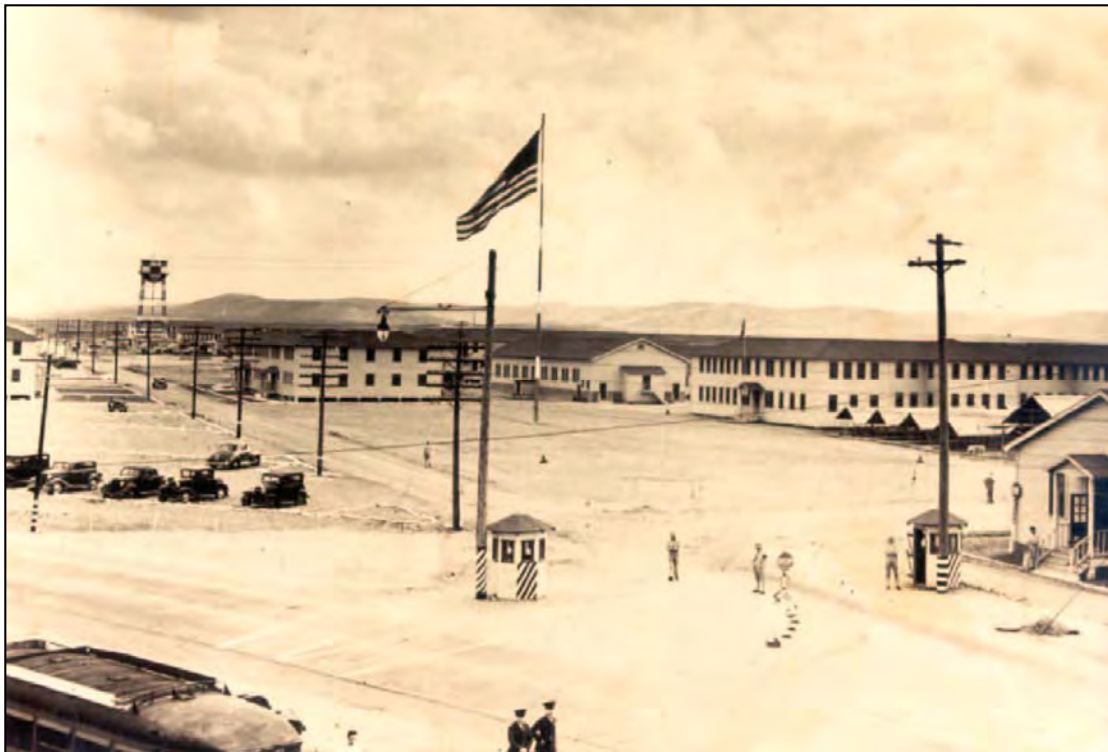
West gate of Camp Elliott from Highway 395 (courtesy of MCRD Museum Historical Society).
